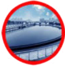
Water & Sewerage Treatment Plants
